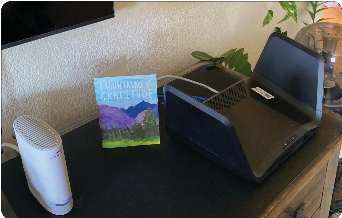
FIG 7. MODEM AND WI-FI ROUTER GROUNDED
